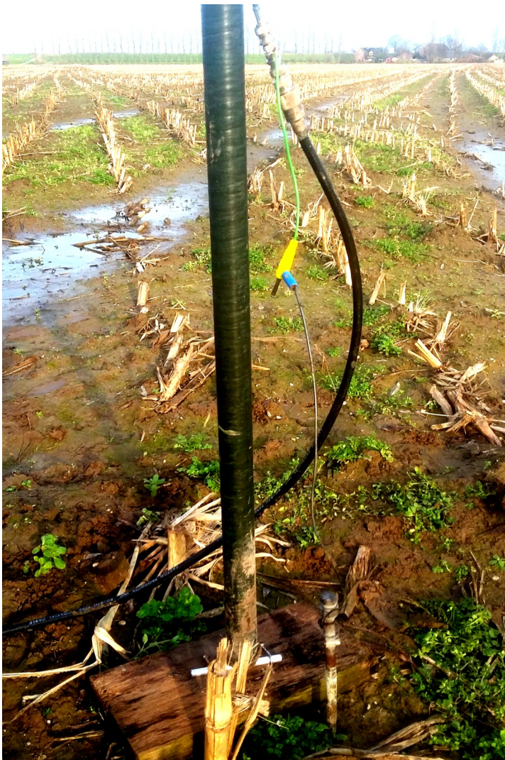
Grounding the antenna is essential for a good reception.
