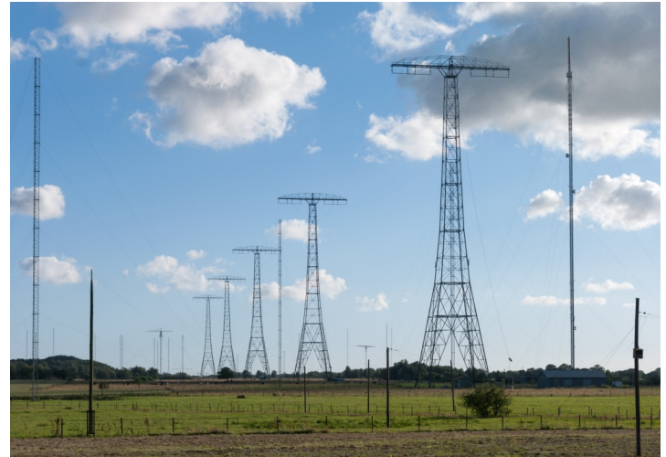
The huge VLF antenna of SAQ near Grimeton, Sweden ( credits ).
